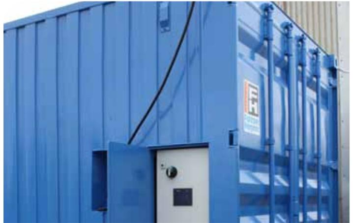
The control panel on the Emo Cube includes an easy to use switch for engaging the pump.
